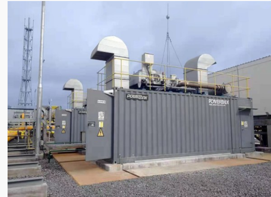
Ghana National Natural Gas Project
