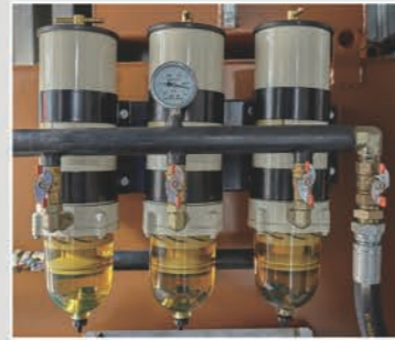
Multi-stage fuel/water separator
